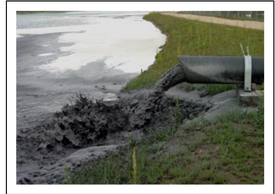
PFA slurry discharging into a lake. This is the fate that awaits Thrupp Lake
